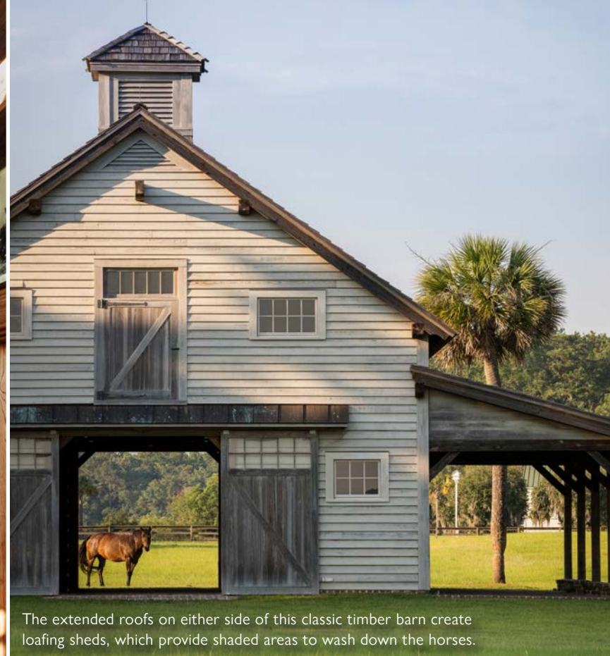
Complete with a brick floor and shepherd's crook sconces, the barn shelters horses, with supporting space for tack and feed.
